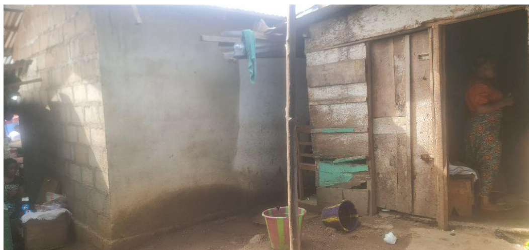
Figure 2-6 Photo of fixed wooden doors privately owned
